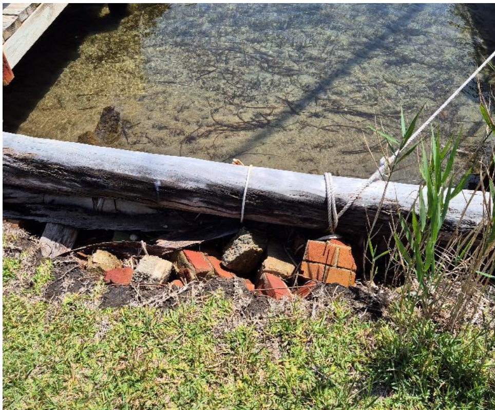
Figure 5-6 Bricks added to fill the scour hole behind the log revetment
