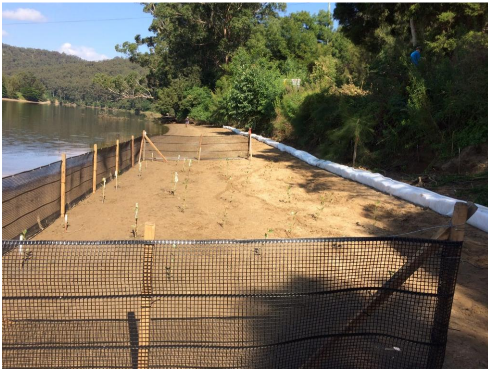
Figure 2-1 Fencing used to shelter mangrove seedlings along Shoalhaven River (Source: Shoalhaven Riverwatch, 2017)
