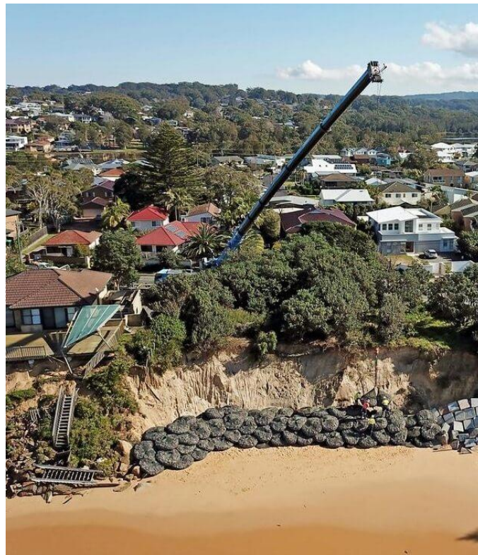
Figure 8-6 Example of rock bags being placed with a long reach boom at Wamberal Beach circa 2020.
