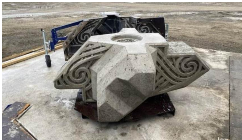
Figure 8-8 Xblock+ armour unit used in New Zealand, incorporating embedded motifs
