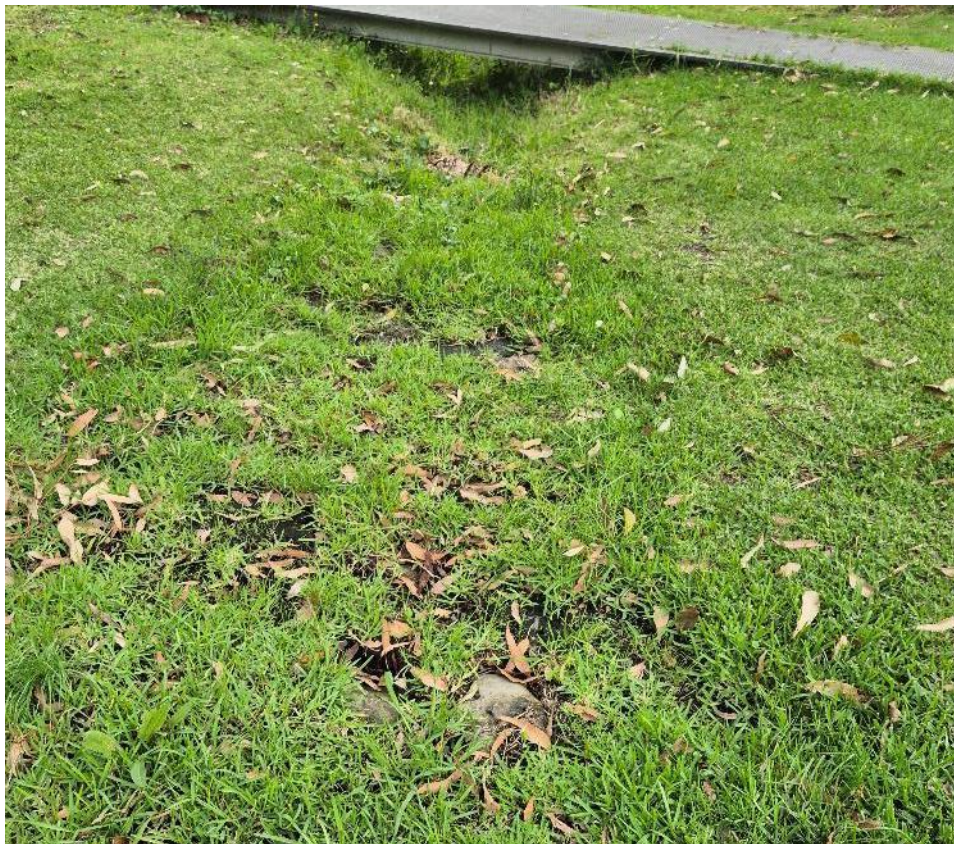
Figure 6-11 Drainage line infilled with rocks (looking downstream)
