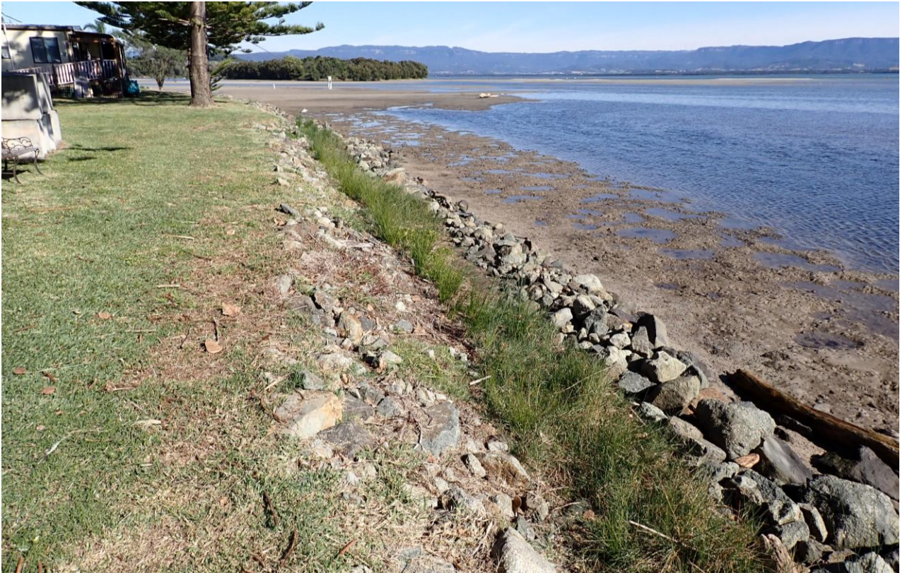
Figure 2-6 Rock fillet work allowing saltmarsh to establish at Lake Illawarra
