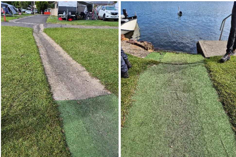
Figure 3-8 Example of Spoon Drain in Reach 3 of Site 1 (Left: Looking away from Lake and Right: Looking towards Lake)
