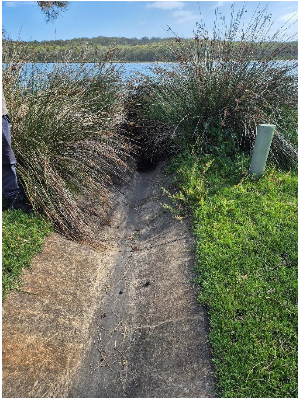
Figure 3-9 Spoon drain terminating at a stormwater pit.
