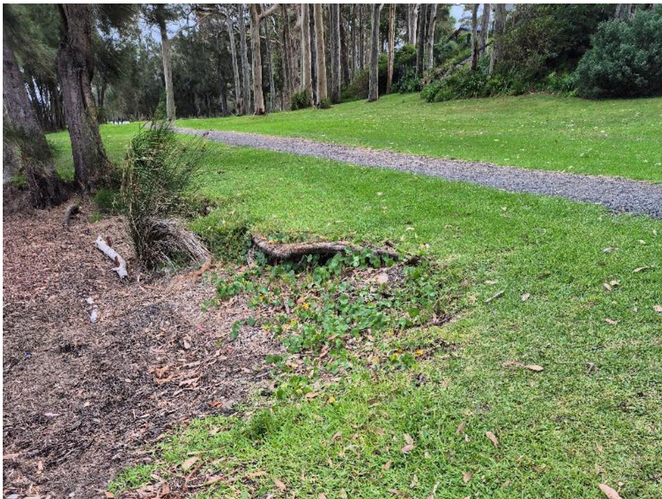
Figure 6-7 Site 3b, Reach 3 – Minor erosion on the foreshore
